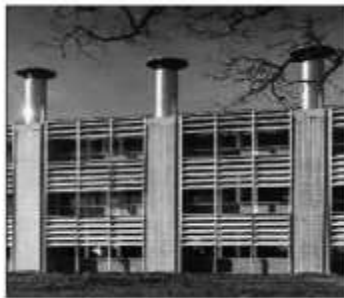
Figure 11 Solar chimney -BRE building
