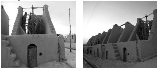
Fig. 9. The edge of the walls have stairways on the south view so that the millers can access different elements and parts of the windmills
