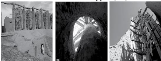
Fig. 4. The wind, passing the wind catcher gate, reached the corners of eight-folded ports and moved the wheel and sails. [ghader agheli]
