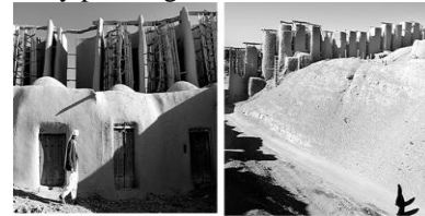
Fig. 7. The Neshtifan windmills are built in a multi-storied form to exploit the wind
