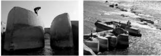
Figure 10. The outer view of the ship foundation which is caulked with gypsum and mortar and filled with mortar
