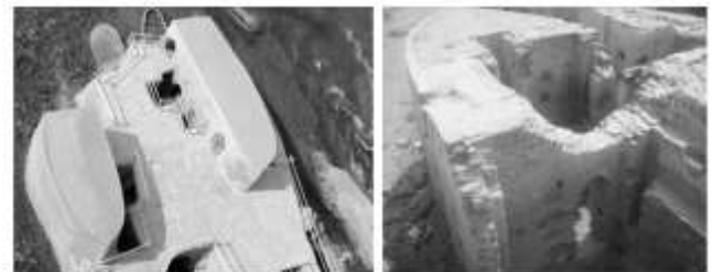
Figure 5. Facade of wave breaker (surfing) nose of Dezful watermills; the watermills of Dezful had a boat-like nose to resist against the formidable tide of Dez River
