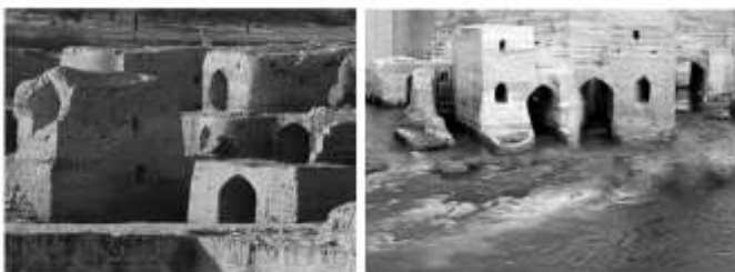
Figure 3. Dezful watermills were built in two floors, of which the first was the place for the installation and the second for grinding the wheat
