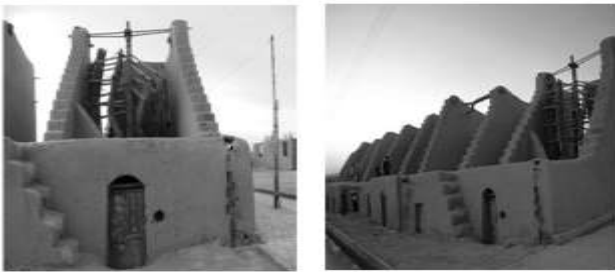
Figure 21. The edges of the walls have stairways on the south view so that the millers can access different elements and parts of the windmills.
