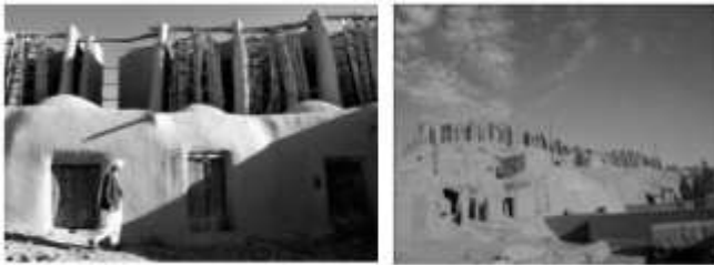
Figure 18. The Neshtifan windmills are built in a multi-storied form to exploit the wind.
