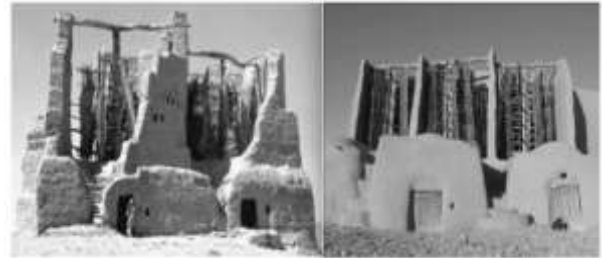
Figure 16. A cylindrical windmill and a simple windmill after restoration
