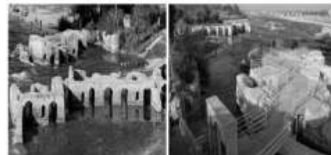
Figure 19. Bridge-watermill of Dezful, spread over the river width successively
