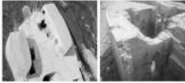
Figure 10. Facade of wave breaker (surfing) nose of Dezful watermills; the watermills of Dezful had a boat-like nose to resist against the formidable tide of Dez River.
