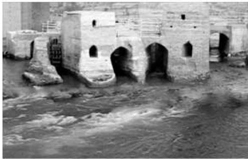
Fig. 4. Dezful watermills are built in two floors. In the lower floor, the installations were located. The upper floor was the place that the grains were ground; [21]
