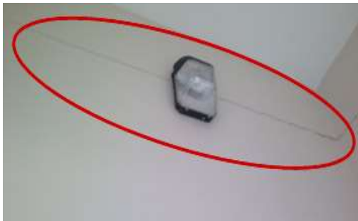
Figure 3: Horizontal cracks at wall on the sides of the light at Hamzah Sendut 3 Library
