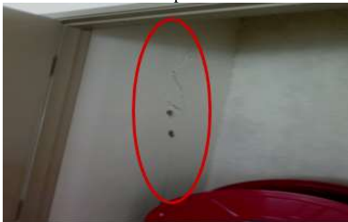
Figure 2: Vertical cracks from the top to the bottom of the wall at Hamzah Sendut 3 Library
