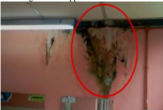
Figure 9: Dampness on wall area at first floor toilet at Aman Damai Hostel
