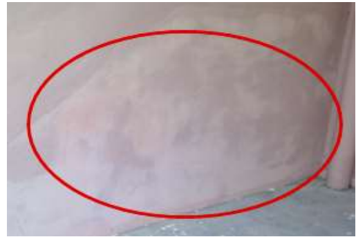
Figure 10: Discolouring on the surface at exterior wall on the first floor at Restu Hostel
