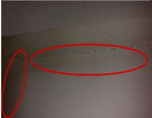
Figure 7: Horizontal and vertical cracks on internal wall at Aman Damai Hostel
