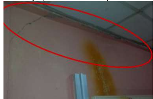
Figure 6: Horizontal cracks at the top corner of the wall at Aman Damai Hostel
