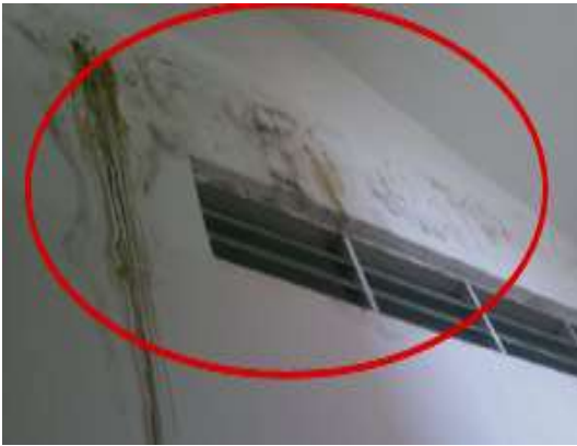
Figure 13: Sign of dampness on wall surface at Restu Hostel
