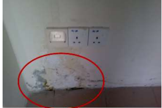
Figure 4: Paint peeling on wall surface at Hamzah Sendut 3 Library
