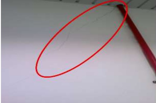
Figure 1: Diagonal cracks on external wall at Hamzah Sendut 3 Library
