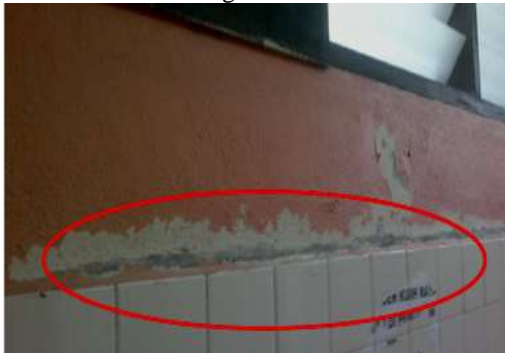
Figure 8: Paint peeling occurred on wall surface in the toilet area at Aman Damai Hostel
