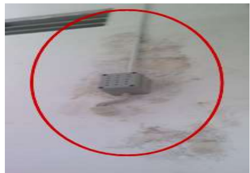
Figure 12: Serious dampness problems at the exterior wall of the toilet at Restu Hostel
