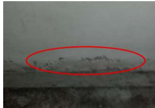
Figure 11: Paint peeling at the bottom of the wall at Restu Hostel
