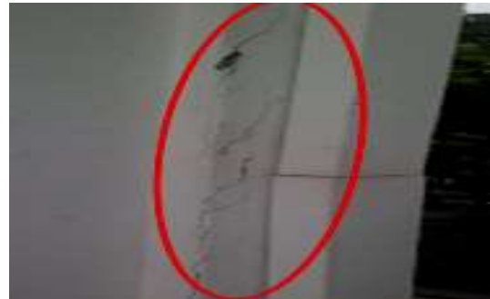
Figure 5: Vertical cracks on the wall surface at Aman Damai Hostel
