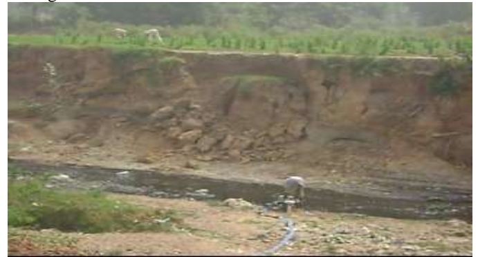
Plate 1 Bank susceptible to erosion and collapse in the Rural Reach of Jakara channel
