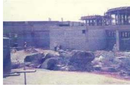
Fig.6 Fly ash bricks used in buildings
