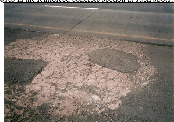
Fig. 1 (c) Figure showing re-occurrence of cracks on the repaired surfaces on a strong stress zone
