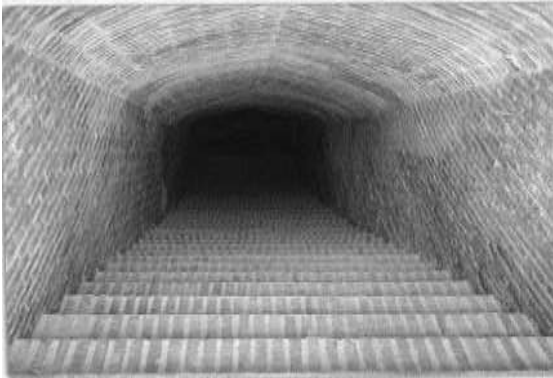
Fig. 22. The above water reservoir was considered as a water supplier for the residents of Lavarestan Town, Fars Province, Iran.
