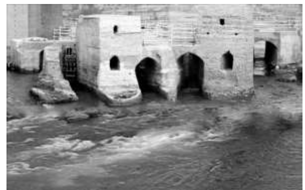
Fig. 19. Dezful watermills are built in two floors. In the lower floor, the installaions were located. The upper floor was the place that the grains were ground. [Author]
