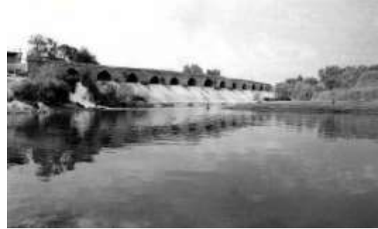
Fig.11. Amir multipurpose dam (Dam, bridge and mill); Age:2000 years.
