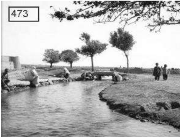
Fig.1. A historic picture remained from 1921 A.D of the watering network of Shah Abdo Al-Azim and Rey Town, between Tehran City and Rey Town.
