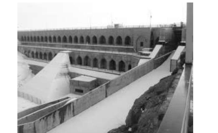
Fig.14. Fariman dam, khorasan Rasavi province, Iran. It has been built on Fariman River and belong to Teimorid dynasty.
