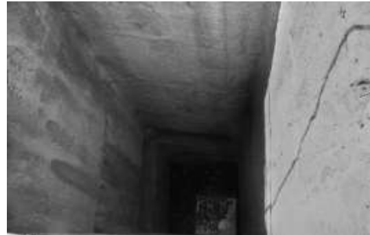
Fig.6. The above hole, which is made of stone, is one of the solutions made by designers of Takht-e-Jamshid structure in order to direct the river outflows [author, 2012].
