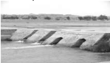
Fig.10. This weir mill divides the Karoun River into two and four branches between Gar Gar and Shatit [author, 2012].
