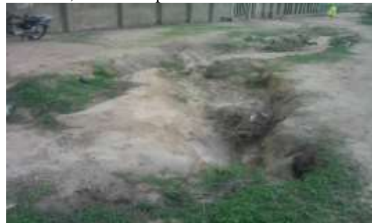
Plate I: This access road has been made almost inaccessible as a result of gully erosion at MTP 90 (Bosso Low Cost Extension)
