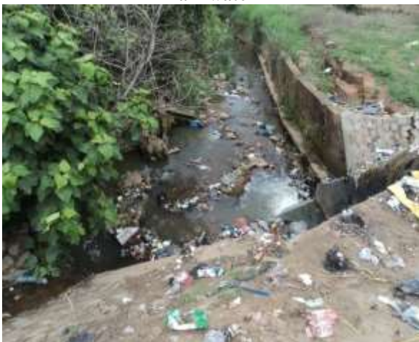
Plate V: an open drainage used as a refuse dump
