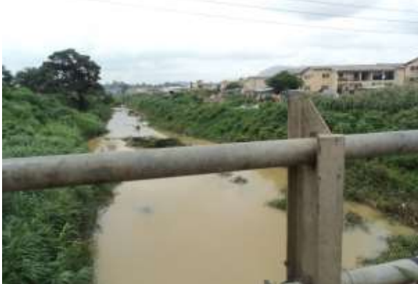
Plate IV: an obstructed canal causing the ponding of excess rain water
