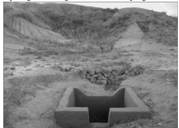
Figure 11. Check dams constructed across the gully of basin area
