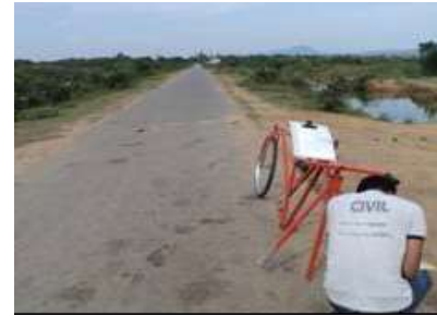
Figure 3. View of Rural Road measuring roughness with MERLIN (W4)
