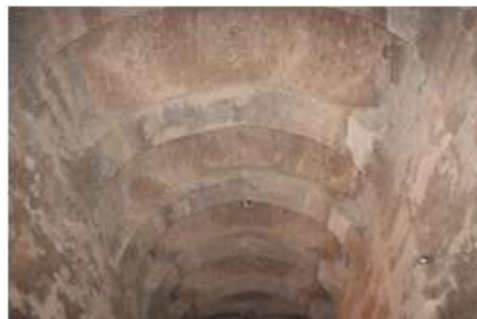
Fig 5. Tagh Kazhave (Barrel-Vault) for Roof cover.
