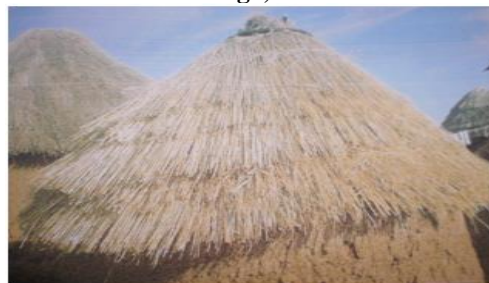
Appendix 2: A building roofed with Phragmites karka at Bontanga, Ghana
