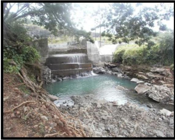
Fig 1. View of damaged tail channel of overflow structure
