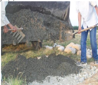
Fig 3(a). Base preparation
