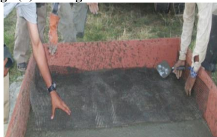
Fig 5(c). Glass grid at 200 mm from bottom.
