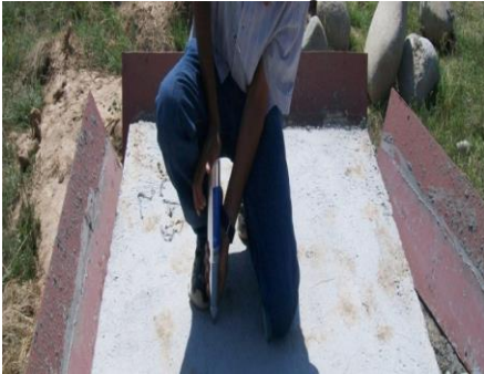
Fig. 6(a). Non destructive test (NDT)
