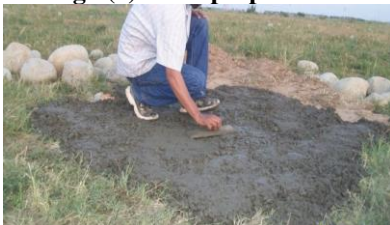
Fig 3(b). PCC of M-15 grade used as cement treated base for the model slabs
