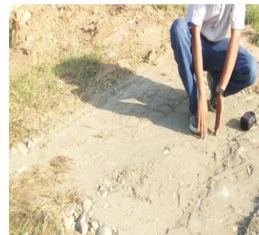
Fig 1.(a) Subbase preparation
