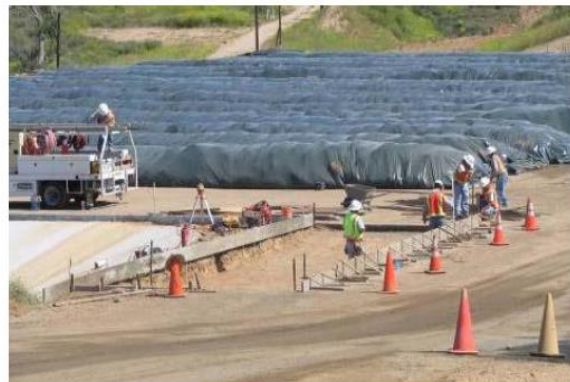
Figure 8. Ex-situ Anaerobic Bioremediation in Bags at an Industrial Site
