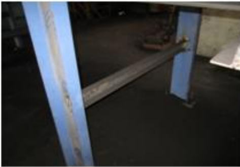
Photograph 3.1. Strengthening of frame structure
