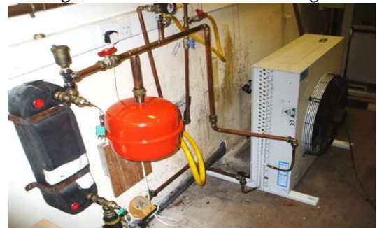
Figure 15. Shows the connections of the heat exchanger, water pump, heat rejection fan and expansion valve.
