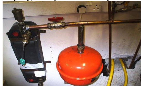
Figure 16. Shows the connections of the heat exchanger and expansion valve.
