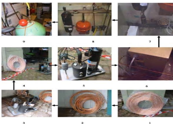
Figure 4. Showing preparation of coils (1-2), installation of heat pump (3-6) and connection of water supply system (water pump, flow metre, expansion valve and the boiler) (7-9).
