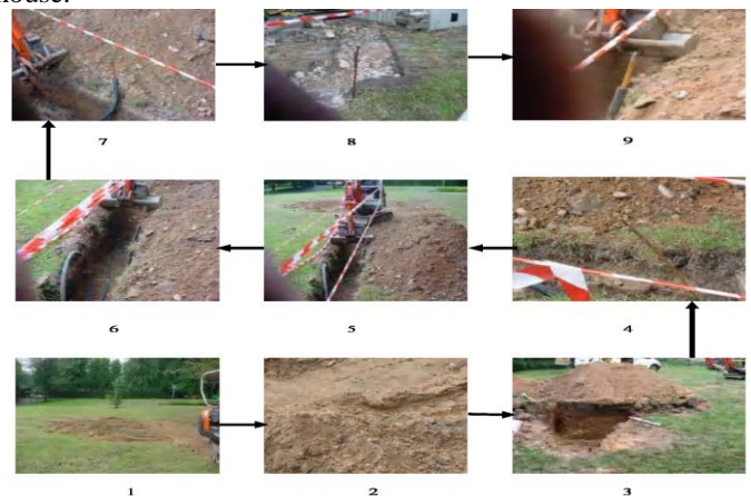
Figure 3. Showing the drilling (1-2) digging of the pit (3), connection of the manifolds (4), grouting, preparation of the coils (5-6) and the source loop, which consists of two earth loops: one for vapour and one for liquid (7-9).
