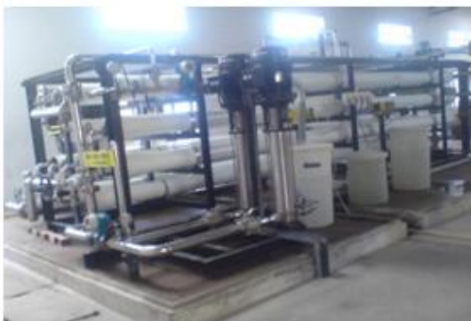
Figure 4 Reverse Osmosis plant 10 Lack liters capacity
