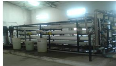
Figure 6 Reverse Osmosis dosing tanks
