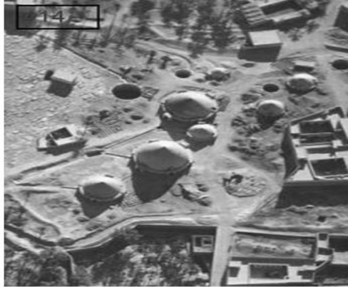
Fig.2. Historic photos of solar water storage, 1970 (Google Earth).
