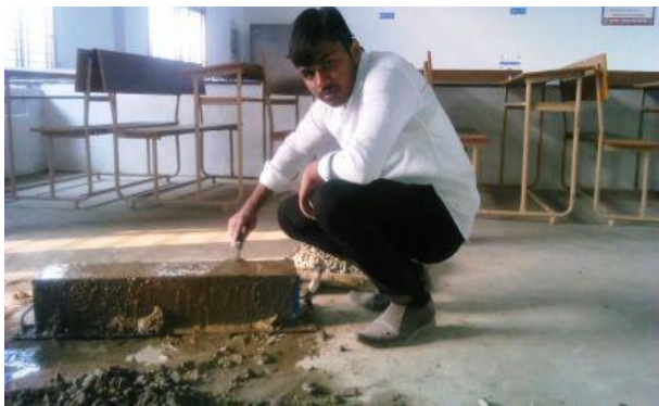
Figure 2. Mixing of materials in 90 kg mixer.
