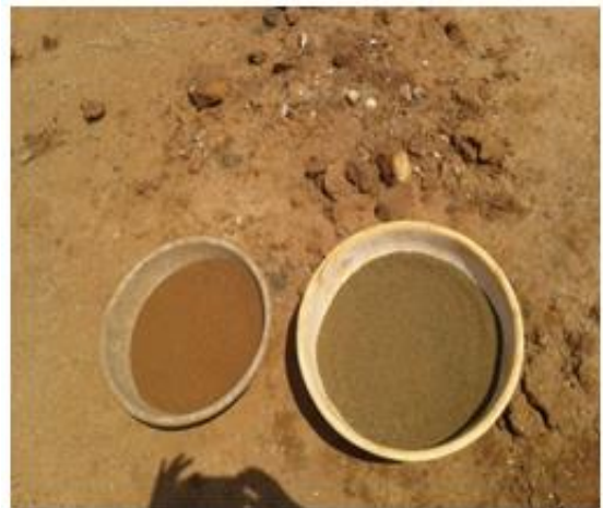
Figure 3. Volume batching.
