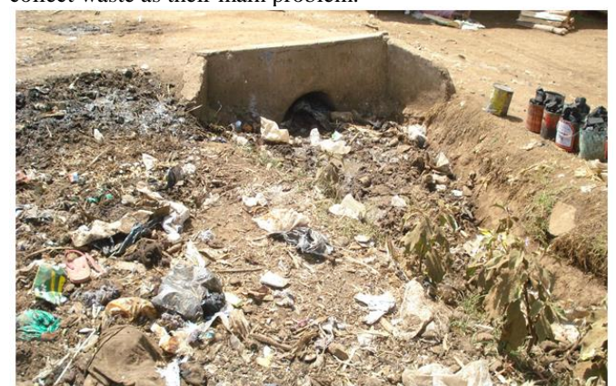
A photo showing storm drainage channels they have become sites for both solid and liquid waste disposal. A photo taken in Langas informal settlement
