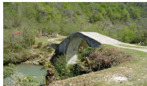
Figure 2. The stone bridge in Varjanauli.
