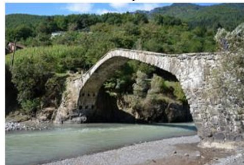
Figure 4. The stone bridge in Dandalo.
