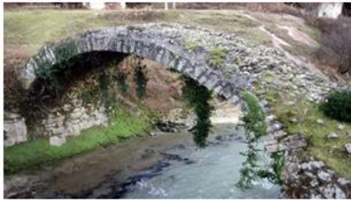
Figure 5. The stone bridge in Tsoniarisi.
