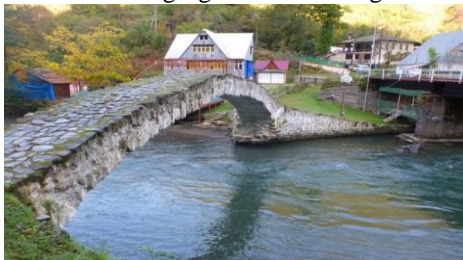
Figure 3. The stone bridge in Machakhela.
