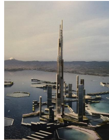
Figure 5.10. NK Sky Tower, Tokyo.
