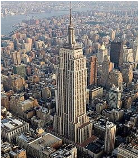
Figure 5.7. Empire State Building, New York.
