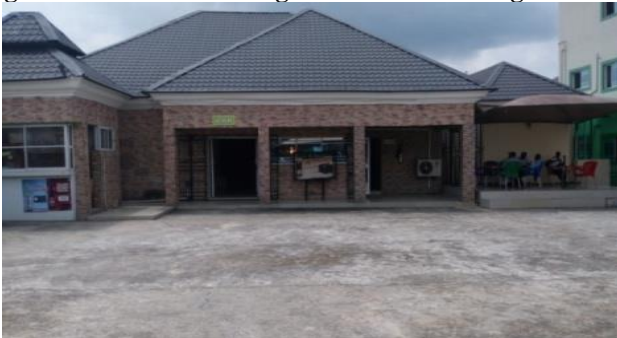
Figure 3. Concrete Building with Unrusted Corrugated Iron Roof.
