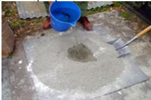
Fig 6 . Water pouring in cement mix.
