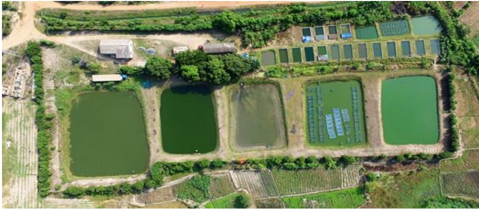
Plate 1. Aerial view of the Aquaculture Demonstration Centre, Ashaiman.
