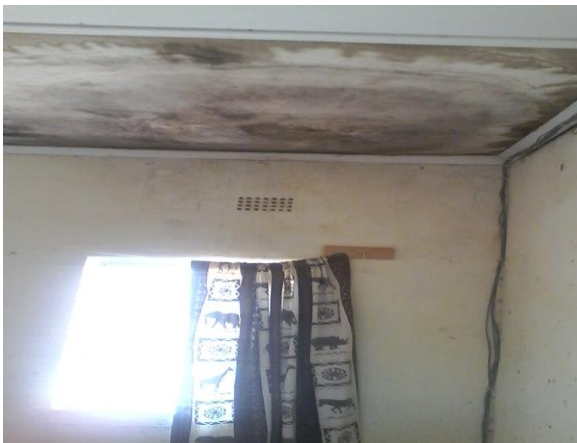
Figure 6. Leaking computer laboratory roof at High School C.
