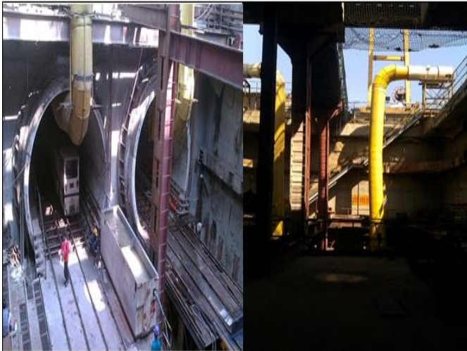
Figure 1. Auxiliary ventilation system via duct during construction of Kolkata metro
